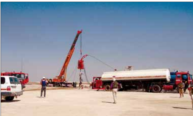
All in a day’s work Above: Crews use acid to open previously made perforations in the oil well to make the resource flow better. The job usually takes one or two days to complete, Capt. Richard Fritzley said. Below: Another part of Fritzley’s job is serving as liaison for the Iraqi media. Questions in Arabic are translated to him in English and then his responses are translated back to Arabic. Submitted photos
