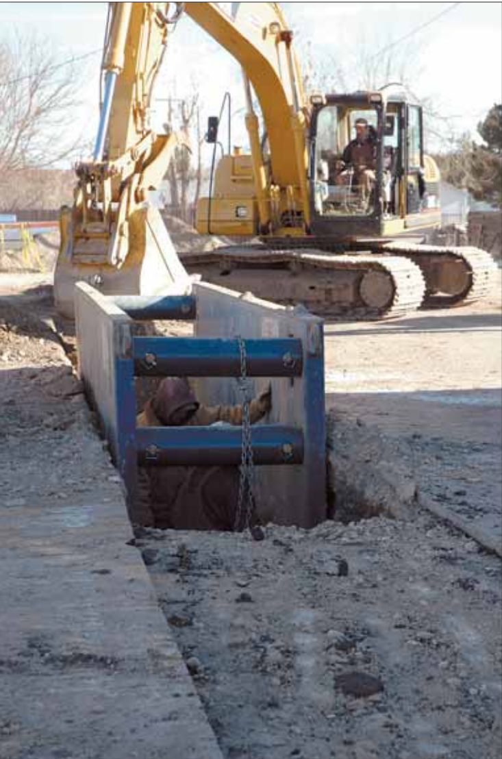
Left: Uria Pump workers Terry Deweese and Mike Riley examine the trench dug by foreman Steve Atkins, background in construction machine, during the early stages of the project in the Paul’s Market parking lot. Above: Project foreman Atkins begins trenching the rest of the parking during the sewer line replacement work last week.
